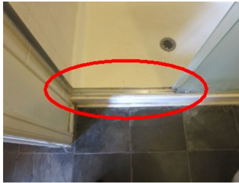
Seal gaps along the master shower
