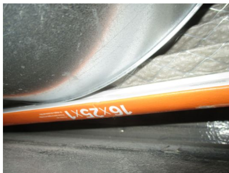
Filter size at time of inspection was 16x25x1
