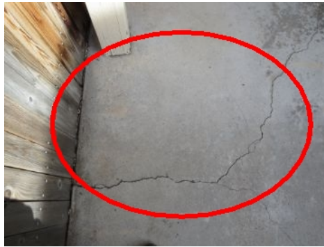
Settlement cracks
