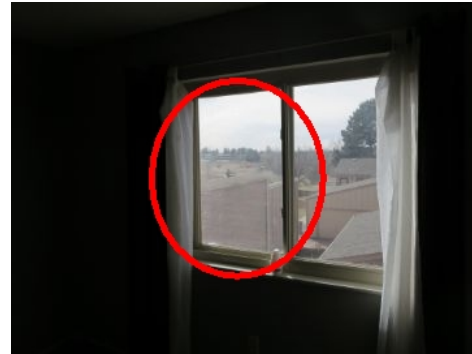
Broken seal in master bedroom window
